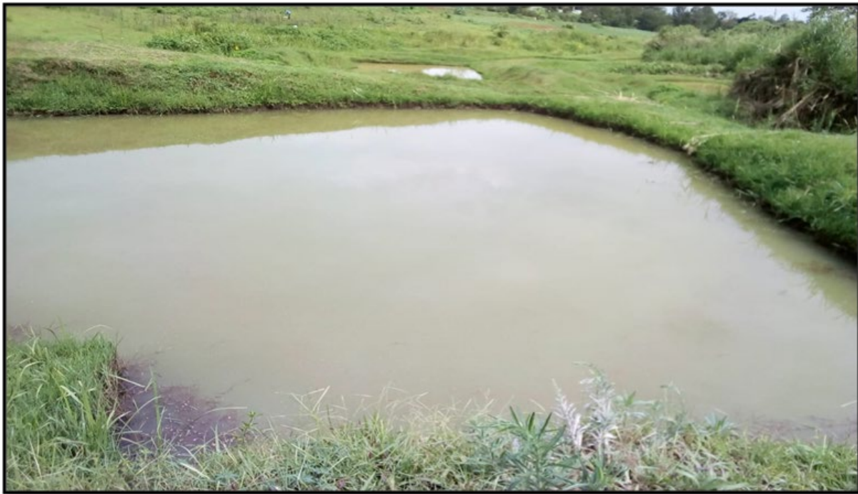
Figure 4: Pond Funded through ESP at Ojolla, South West Kisumu Ward
