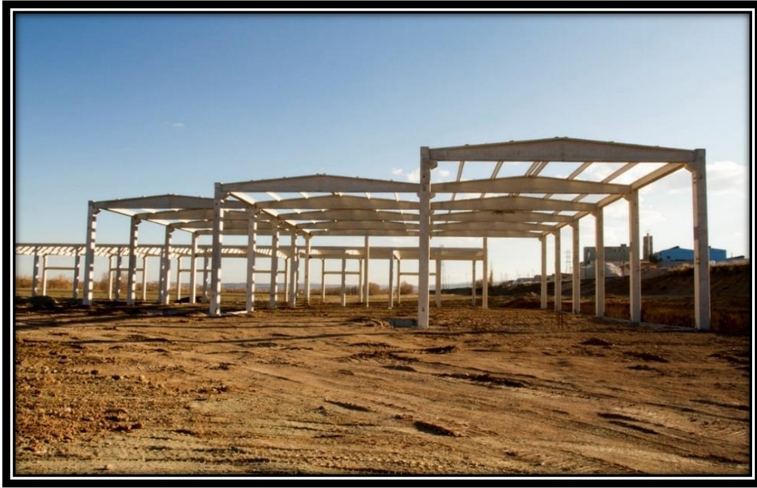
Figure 2: Example of a Concrete Prefabricated Building
