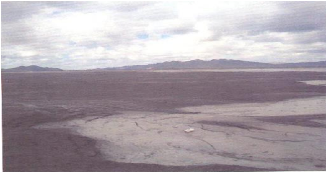
Figure 1: Ash Pond of Mongolian Fourth Thermal Power Plant
