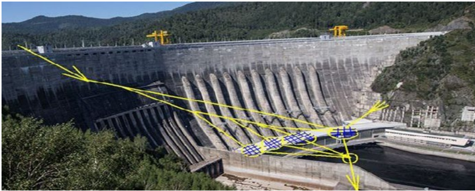
Figure 4: Sayano-Shushenskaya HPP Crossed by HC channels
