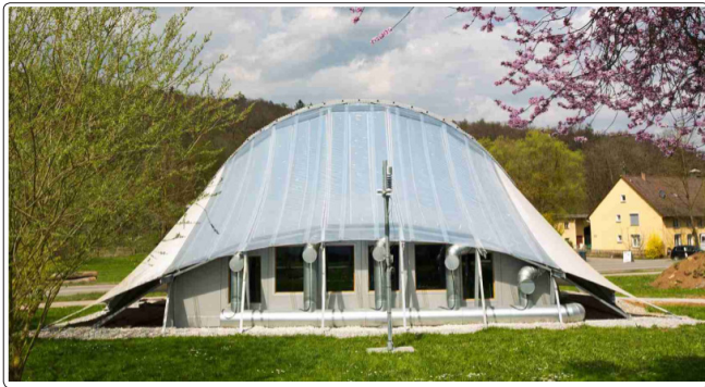
Figure 4: Polar Bear Pavilion with Solar Thermal Roof and Integrated Thermal Energy Storage
