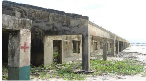
Plate 4a: Former ItakAbasi Primary School located at updrift shoreline damaged by storm surge incident in 2011. Photo: September 28, 2013 (Udo-Akuaibit, 2013).
