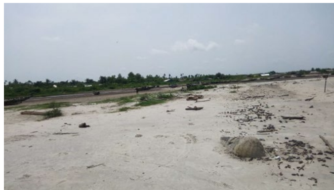
Plate 3b: Severe erosion at updrift estuarine shoreline. Photo: March 17, 2024.
