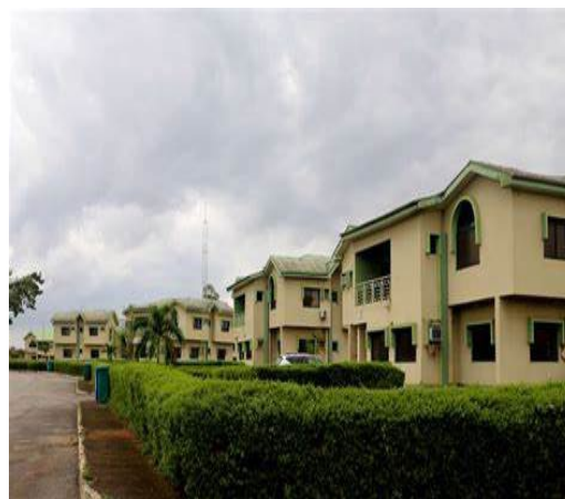
Figure 7: Showing the Gable Roof used at Covenant University Ota, Nigeria Source:- (Covenant University, 2021) [13]
