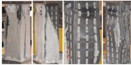
Figure 2: Stages of Crack Development; cover spalling; longitudinal steel buckling and transverse steel fracture; and final failure of the Specimen [10].
