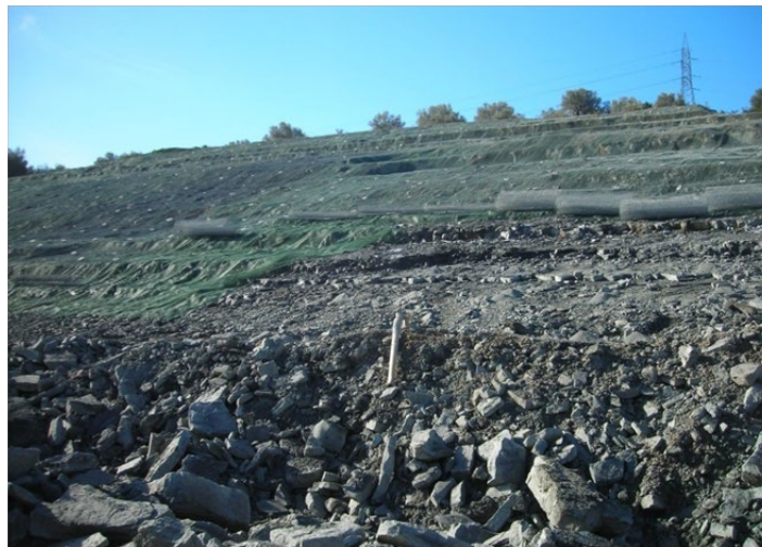
Figure 6: Double Stabilizing Sheet: Bio-Geogrid + Wire Mesh on a Fractured Rock Slope.
