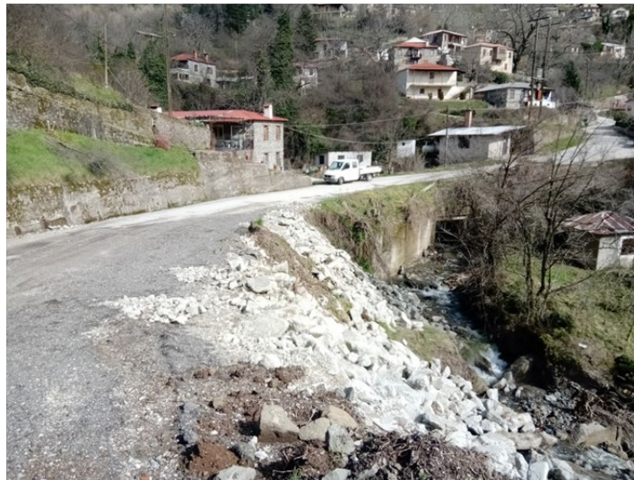
Figure 8: Staged Reconstruction of Damaged Road for Improved Safety
