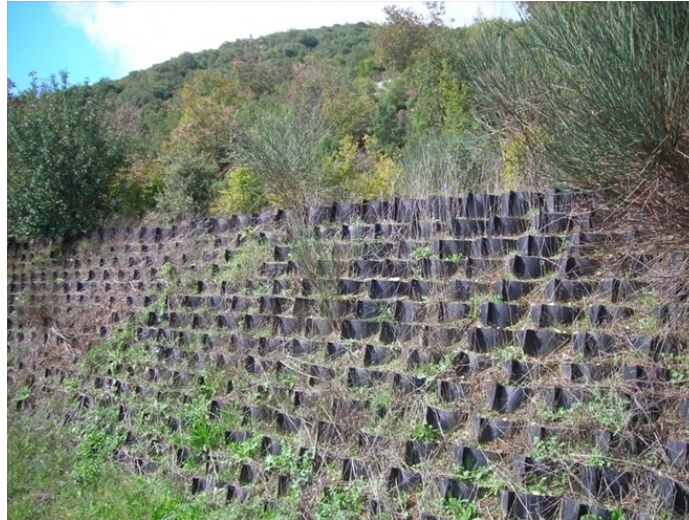
Figure 5: Geocells on Cut Slope for Stability Improvement
